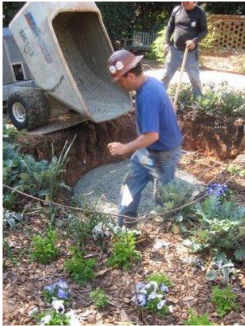
Motorized wheelbarrows will be used to move materials
